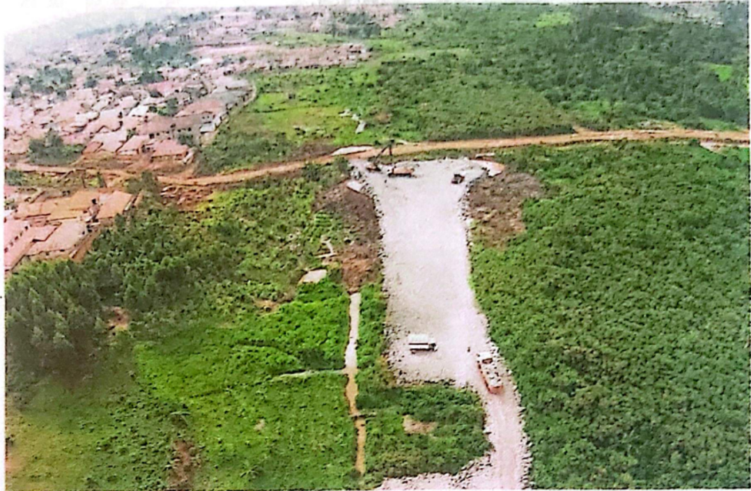
The roadworks at a swampy section of the Busega-Mpigi Expressway in Kyengera Town Council. The resumption of works on the road marks a tangible step forward after years of interruptions. PHOTO/ SADAT MBOGO
