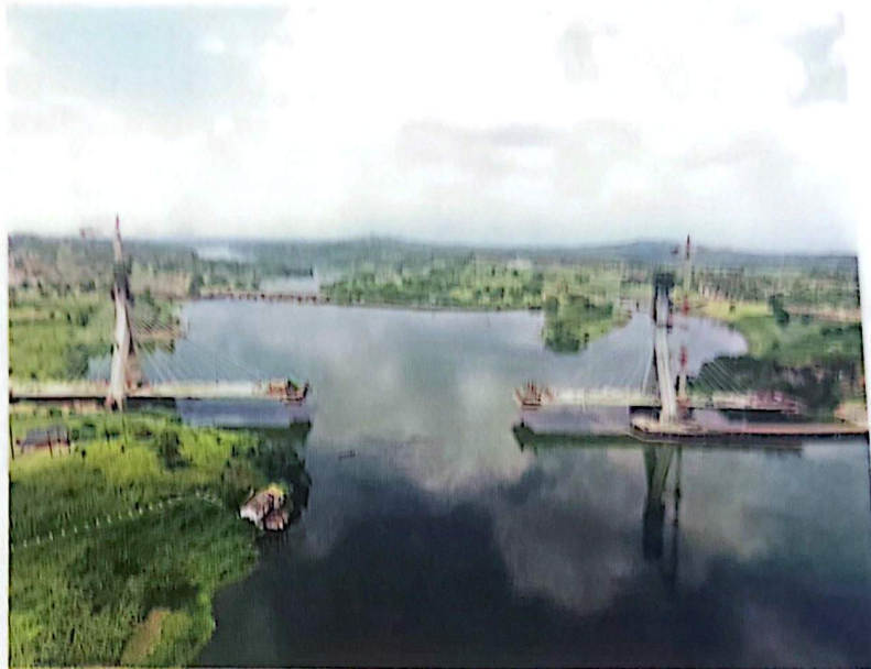
The new bridge has design features that allow for faster flow of both cargo and regular traffic, with two traffic lanes and two walk-ways. It has a design speed of 120km per hour
