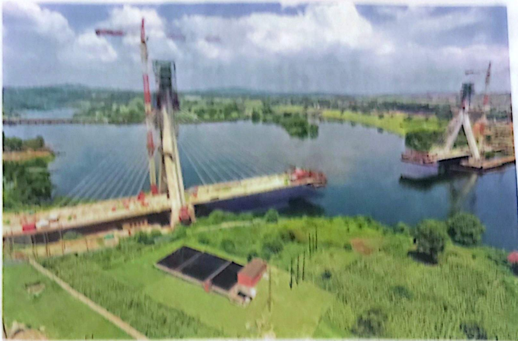
The bridge is expected to be complete next year and will also serve as a tourist attraction because of its uniqueness
