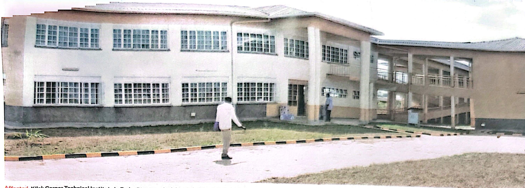
Affected. Kilak Corner Technical Institute in Pader District which has failed to attract students. PHOTO BY TOBBIAS JOLLY
