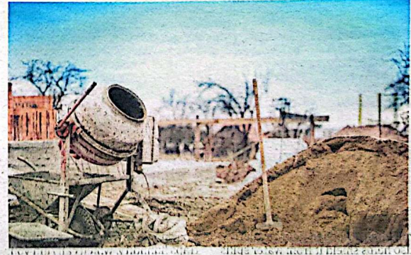
Sand is mixed with cement and stones to give the mortar or concrete mix the structural strength it requires.
