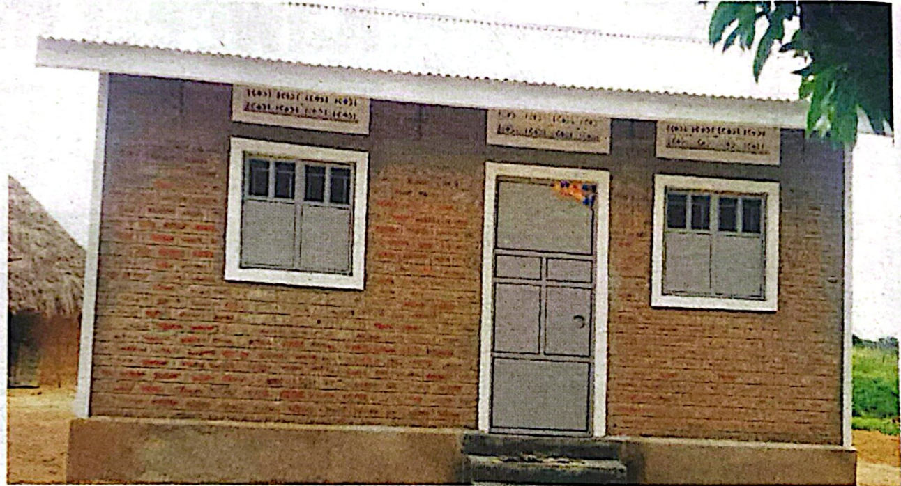
One of the houses that were built for the locals in Kumi district. Photo by Stella Naigino
