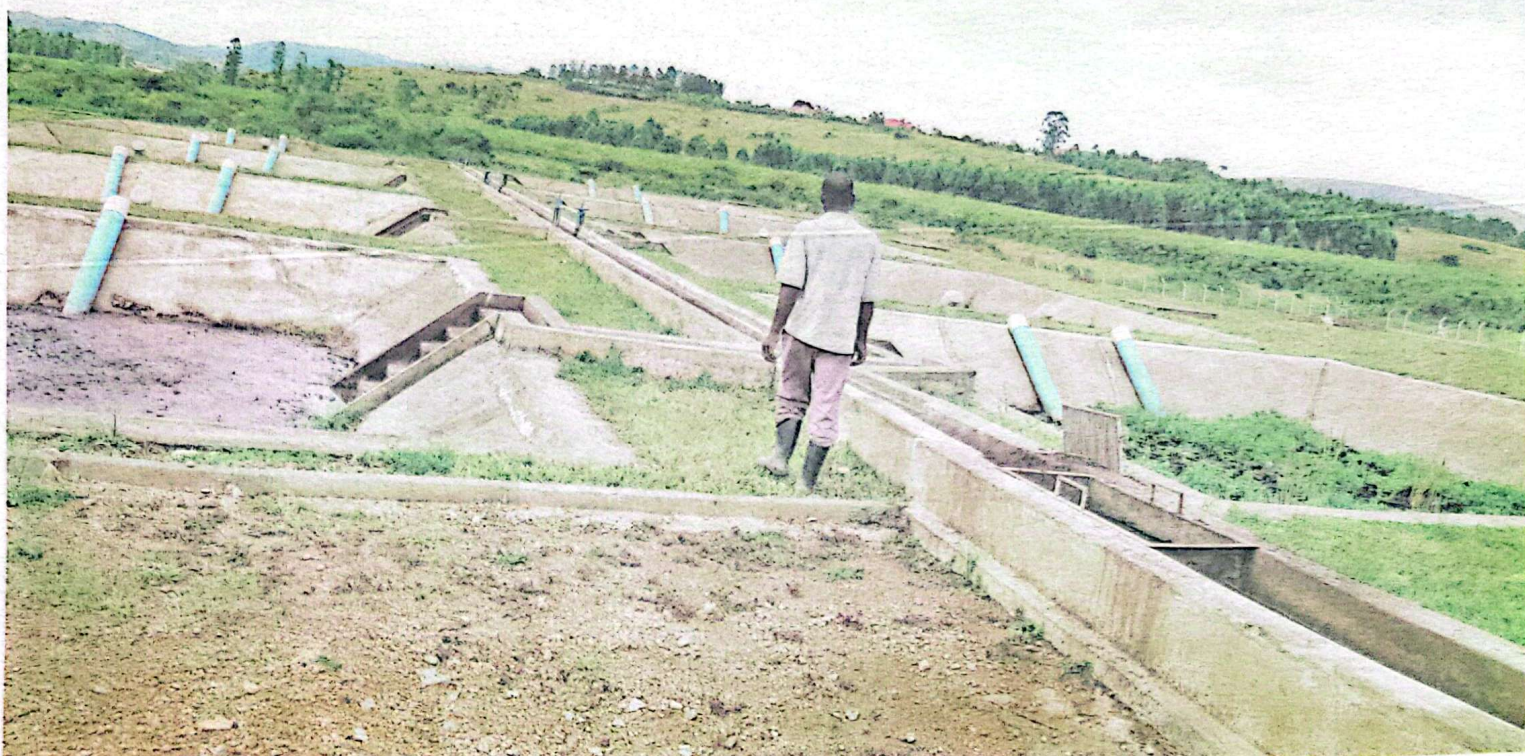
Idle. The faecal sludge that was built under the Lake Victoria Water and Sanitation project has not been used since November last year. PHOTO BY PEREZ RUMANZI
