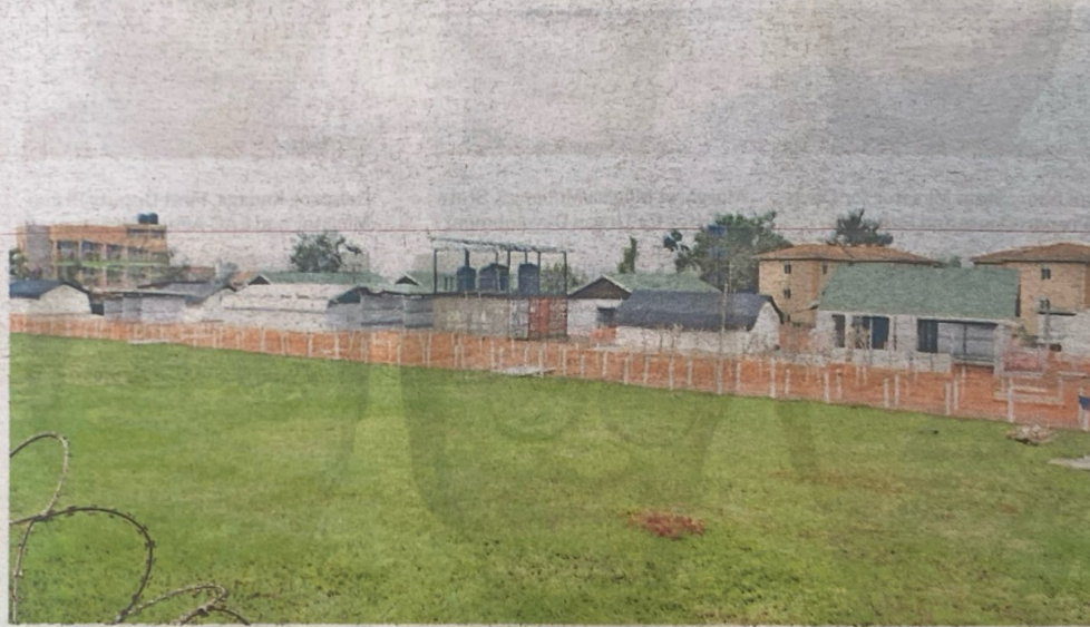
Some of the temporary facilities, which have been constructed at the former Mulago playground to isolate suspected Ebola patients. PHOTO/ STEPHEN OTAGE
