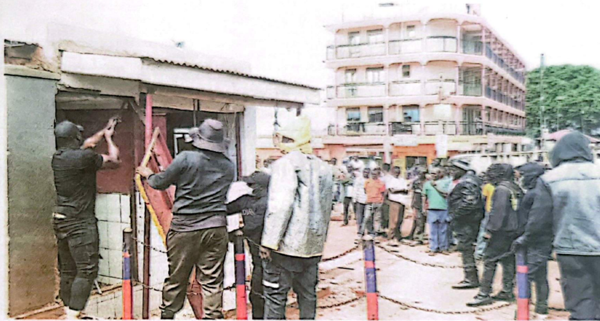
An enforcement team from Mbale City demolish a butcher shop on Bugwere Road Market in Industrial City Division last week. The authorities claim the structures were constructed illegally. PHOTO/YAHUDU KITUNZI
