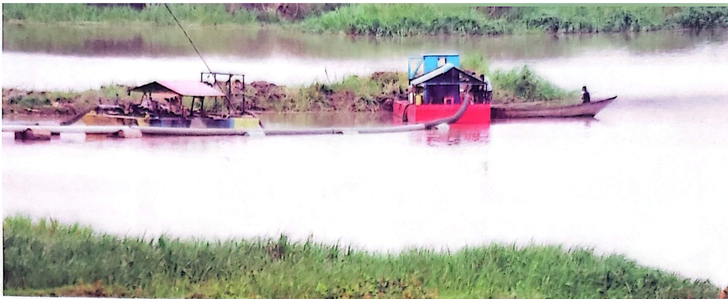
On duty. One of the sand mining sites operated by Porch Group at at Bukolwa village, Nkumba Parish in Katabi Town Council, Entebbe Municipality. PHOTO BY JOSEPH KIGGUNDU
