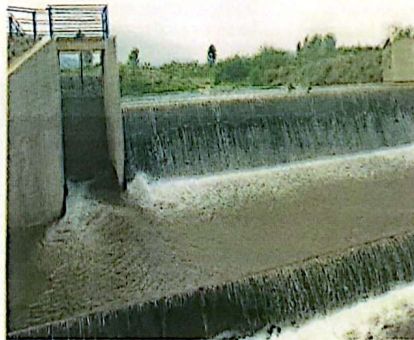
The 14MW Bugoye dam on River Mubuku
