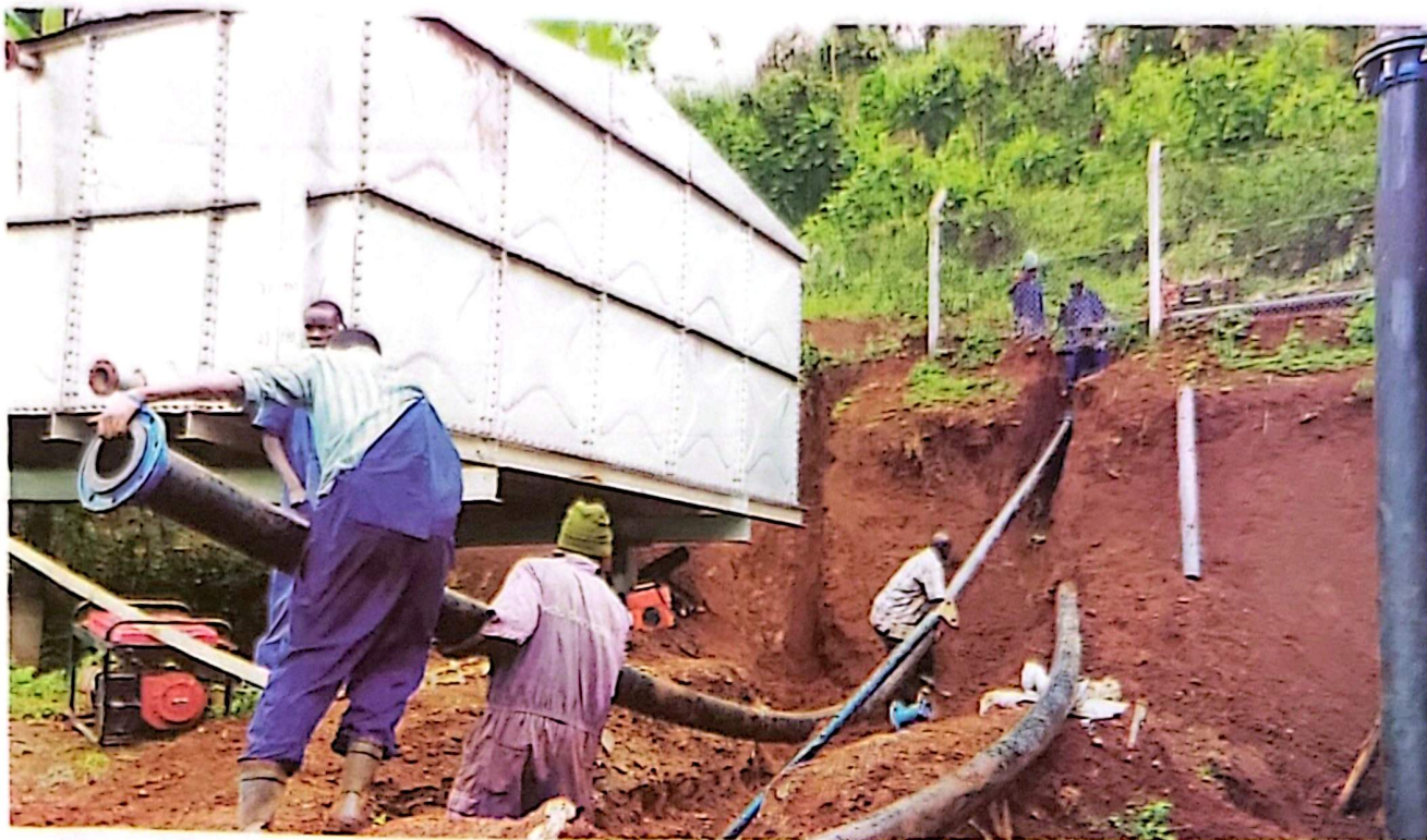
Work in progress Workers connect pipes for the Bududa-Nabweya Gravity Water Flow Scheme recently. (PHOTO BY LEONARD MUKOOL)
