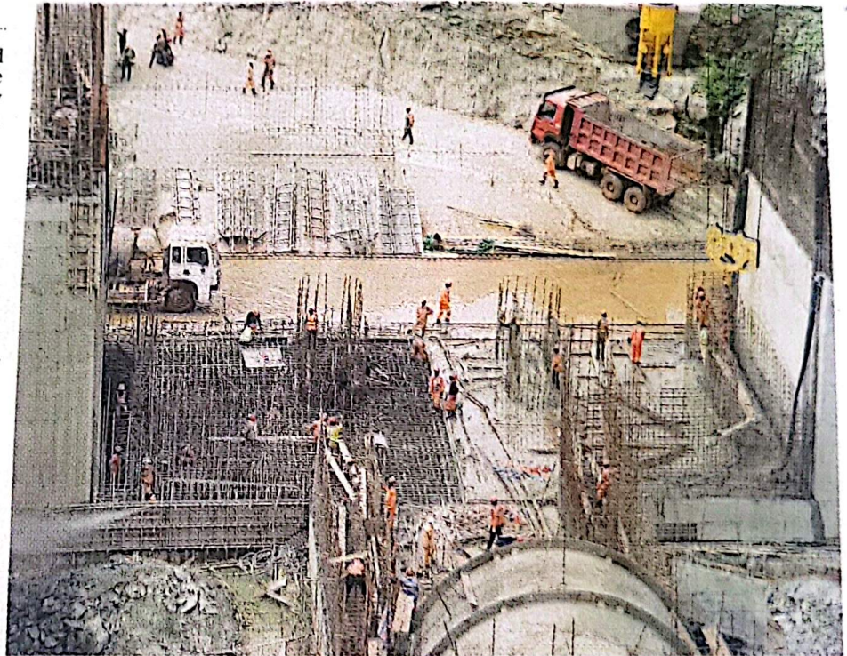
Pressure shafts under construction at Karuma Hydropower project and interconnection transmission line. Uganda has prioritised infrastructure development
