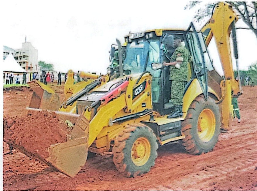
Bulldozers grading the site where a sh5b ICT innovation hub will be built by the army's engineering brigade in Nakawa, Kampala. Photo by Shamim Saad
