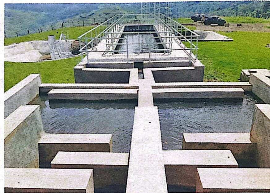
Bukwo water treatment plant in Bukwo district
