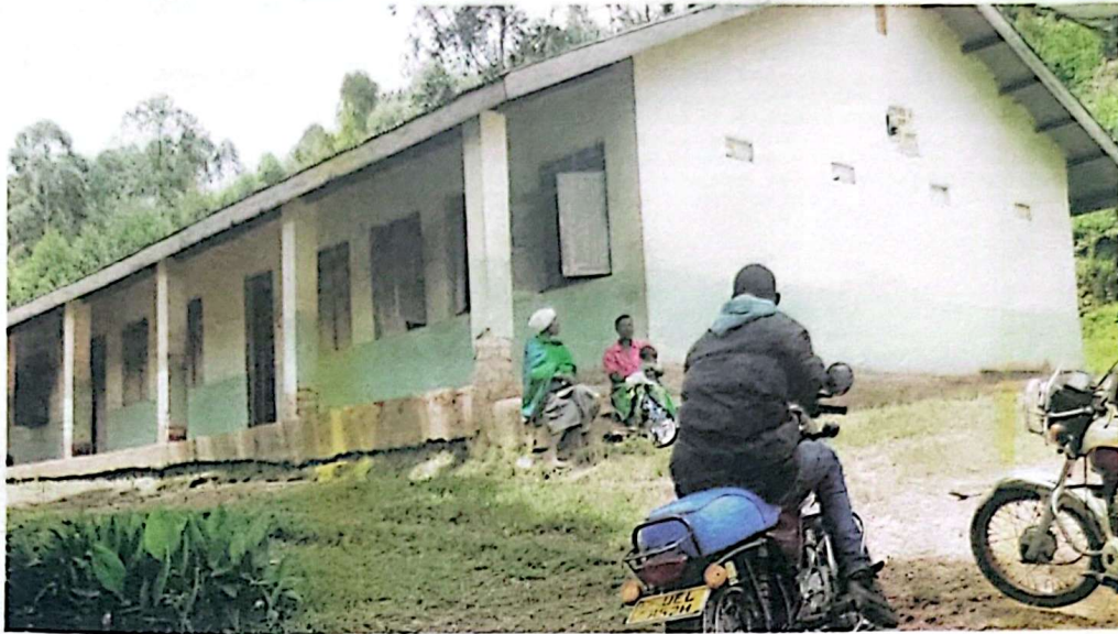
Deplorable. Bwindi Health Centre III building that houses a health centre, sub-county offices and a police post. PHOTO BY ROBERT MUHEREZA
