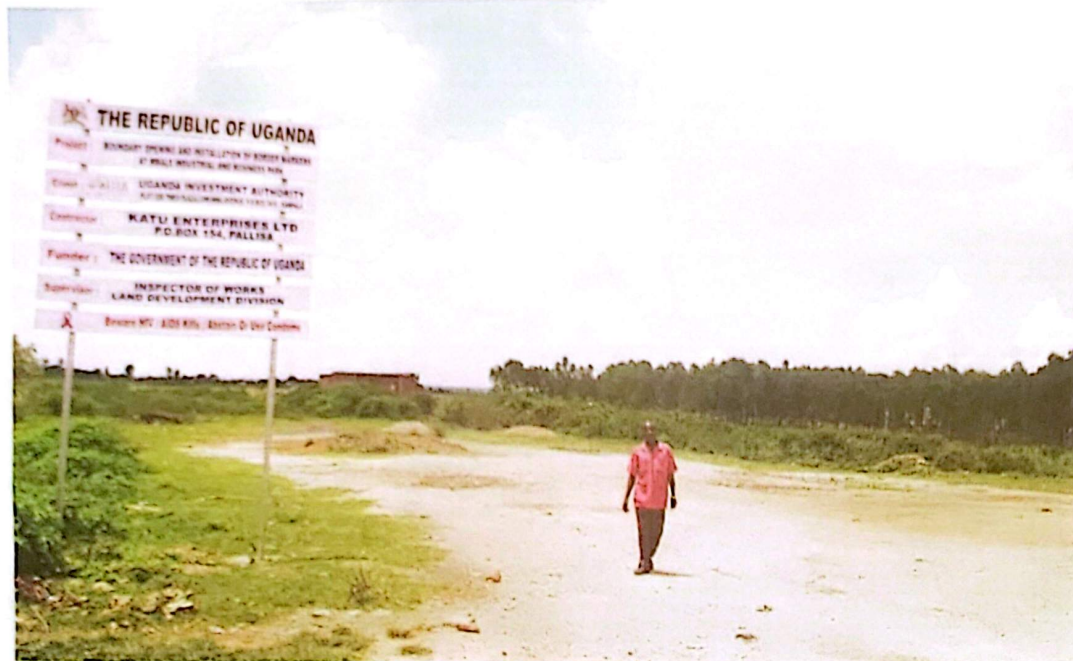
Delayed. Part of the industrial park in Doko Village in Bukasakye Sub-county. Some of the affected residents claim they have not been compensated in order to vacate their land. PHOTO BY FRED WAMBEDE
