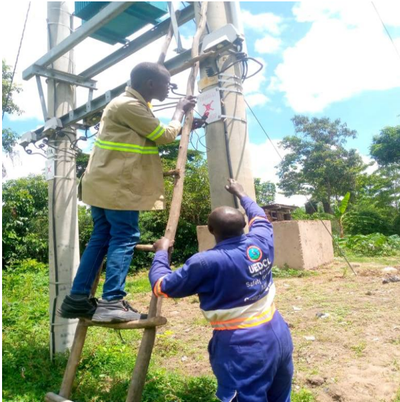
Figure 6: Current measurement on different phases
