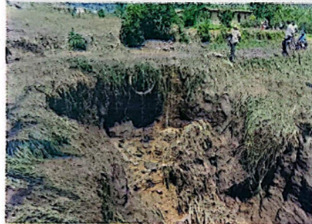
Some of the damage caused by the downpour
