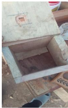
Figure 3. 1: Construction of the frame
