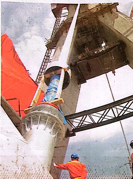
Support structure. One of the pylons of the New Nile Bridge
