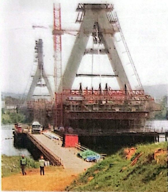
Almost done. Construction of the bridge commenced in 2014.
