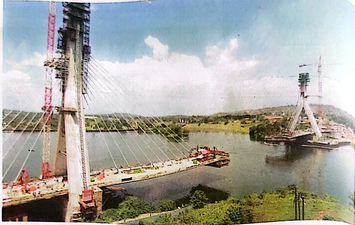
Mega project. Zenitaka Corporation of Japan and Hyundai Engineering and Construction Company from South Korea are constructing the New Jinja Nile Bridge across the Nile river. PHOTOS BY ABUBAKER LUDOWA
