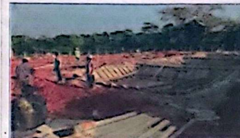
Fecal sludge treatment plant in Kamuli, construction ongoing
