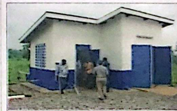
Pumphouse in Kaliro TC
