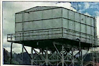
Reservoir Tank for Nakapiripit TC
