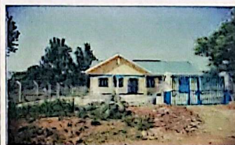
Modern Office block for O&M in Nakapiripit
