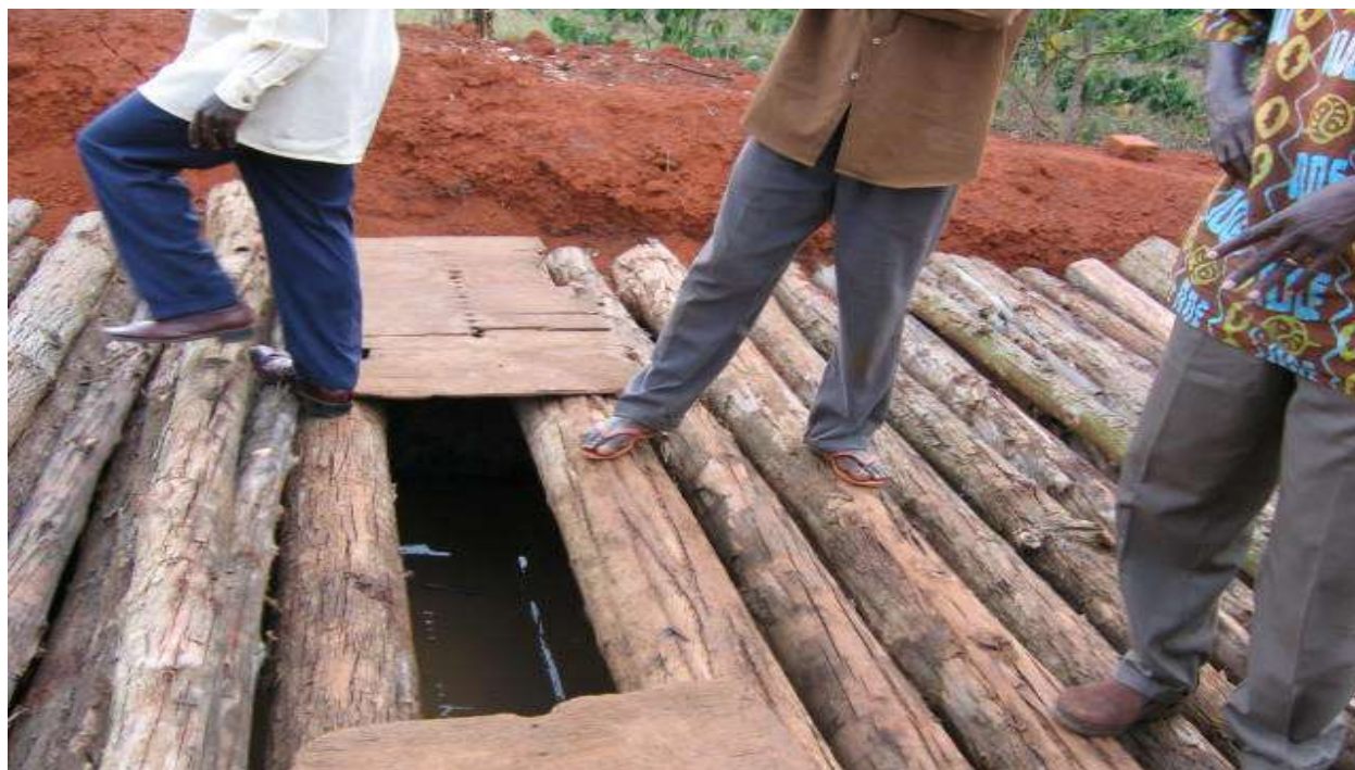
Construction of underground water reservoir
