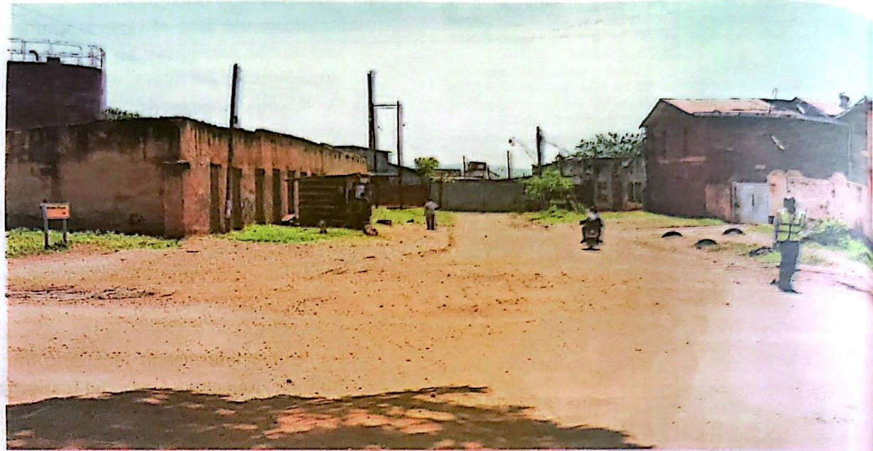
Kisiki, one of the roads in Jinja that was closed after an investor constructed a factory in the middle of it. PHOTO: TAUO NAKATO
