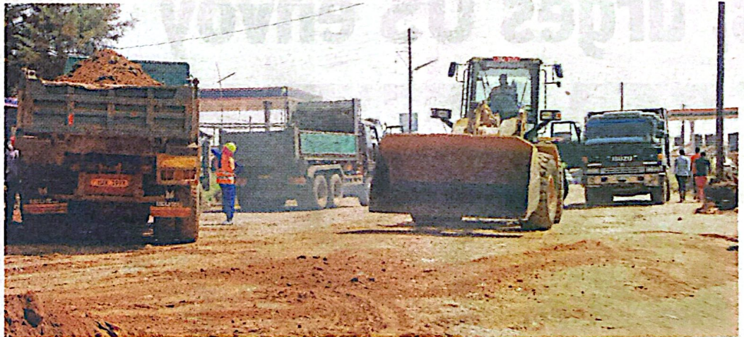
Construction works ongoing on Kwebiiha Road in Hoima town. Photo by Robert Atuhairwe
