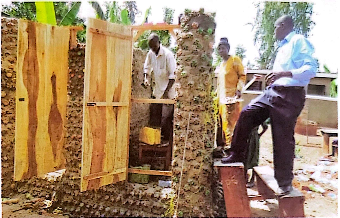
New. Members of Butakoola Village Association for Development construct a pit latrine using bottle-brick technology at Nawandagala Primary School. PHOTO BY FRED MUZAALA
