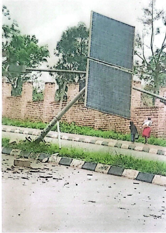
Residents walk past a solar streetlight that was destroyed on Yellow Knife Road in Masaka City last year. Criminals have been exploiting darkness in many urban centres to execute their missions. PHOTO/FILE
