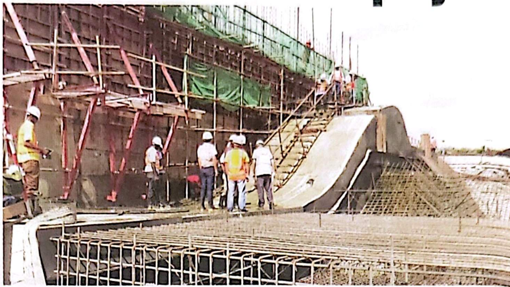
Progress. Engineers at Karuma power dam inspect the ongoing construction recently. PHOTO BY STEPHEN OTAGE
