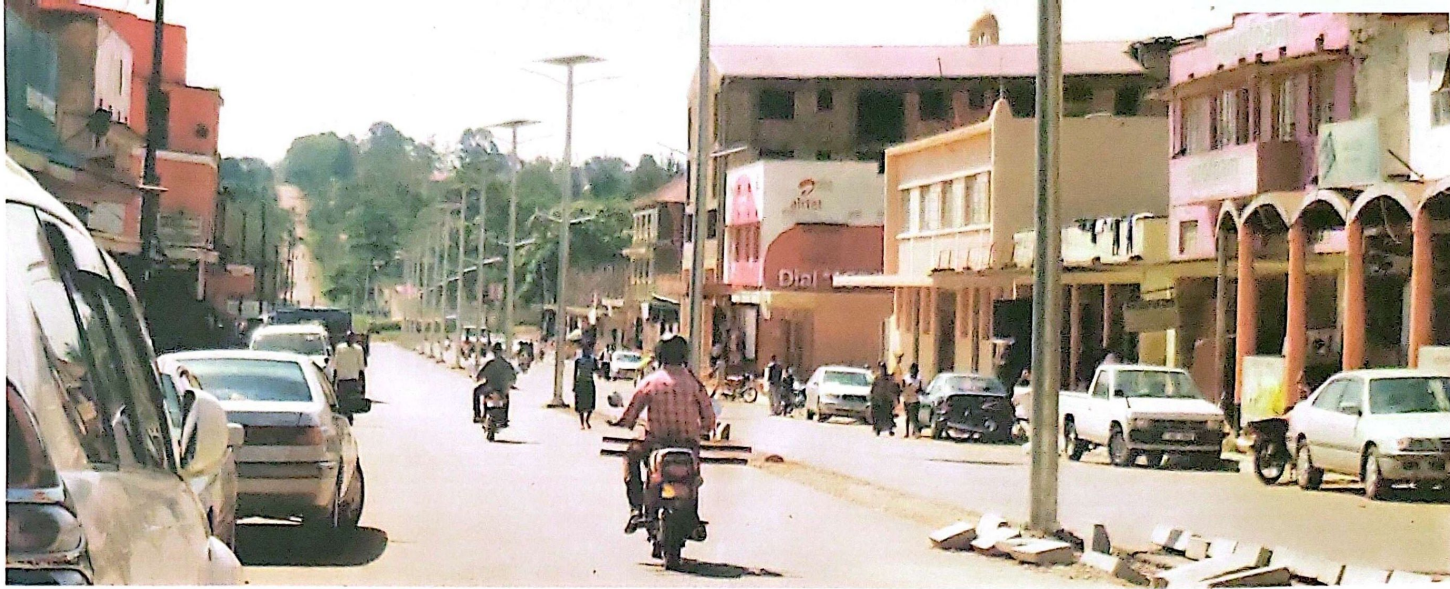
Installed. Solar street lights that have been installed on Edward Avenue in Masaka Municipality. PHOTO BY ALI MAMBULE
