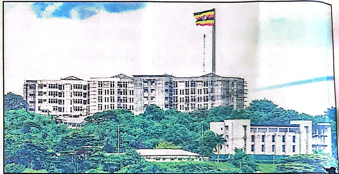
New UPDF headquarters on Mbuya hill in Kampala nears completion, construction hits 75% complete
