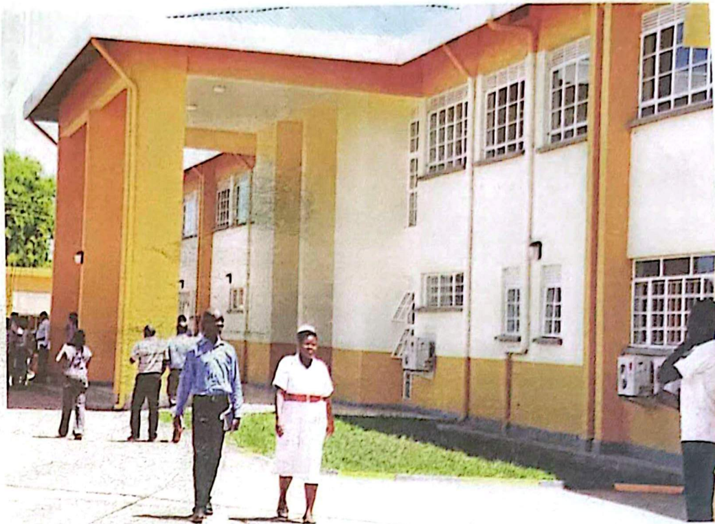
Worst. The recently constructed outpatient department at Moroto Regional Referral Hospital. The hospital has been ranked among the worst performers in a new report. PHOTO BY STEVEN ARIONG
