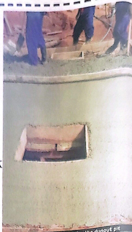
Fill the tank with water before backfilling the dugout pit
