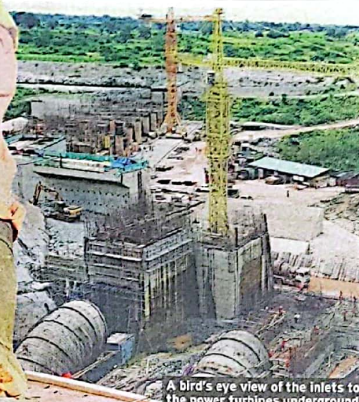
A bird's eye view of the inlets to the power turbines underground
