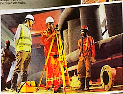
Engineers take measurements for the turbine placement in the powerhouse
