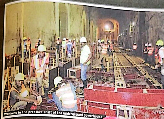
Workers in the pressure shaft of the underground powerhouse
