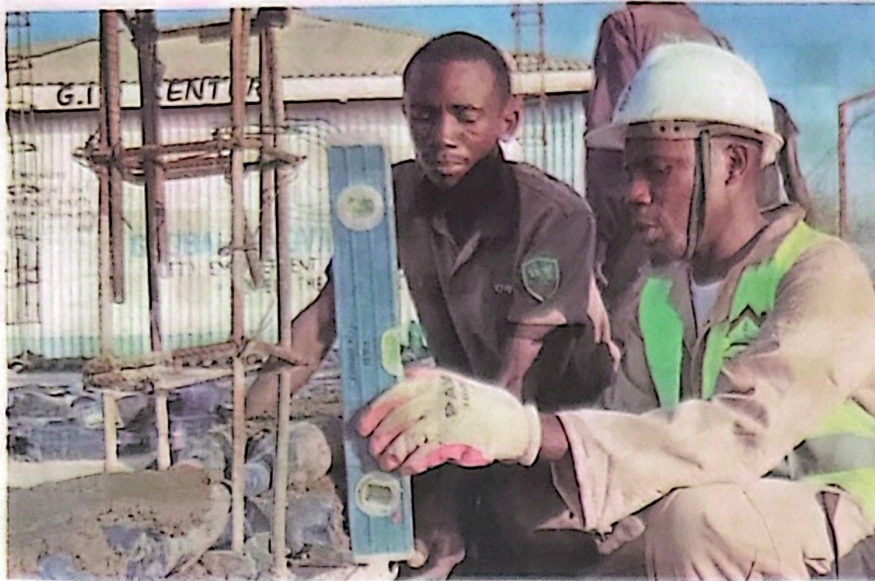
David Monday on a site. His firm constructed the first plastic bottle house in 2014.
