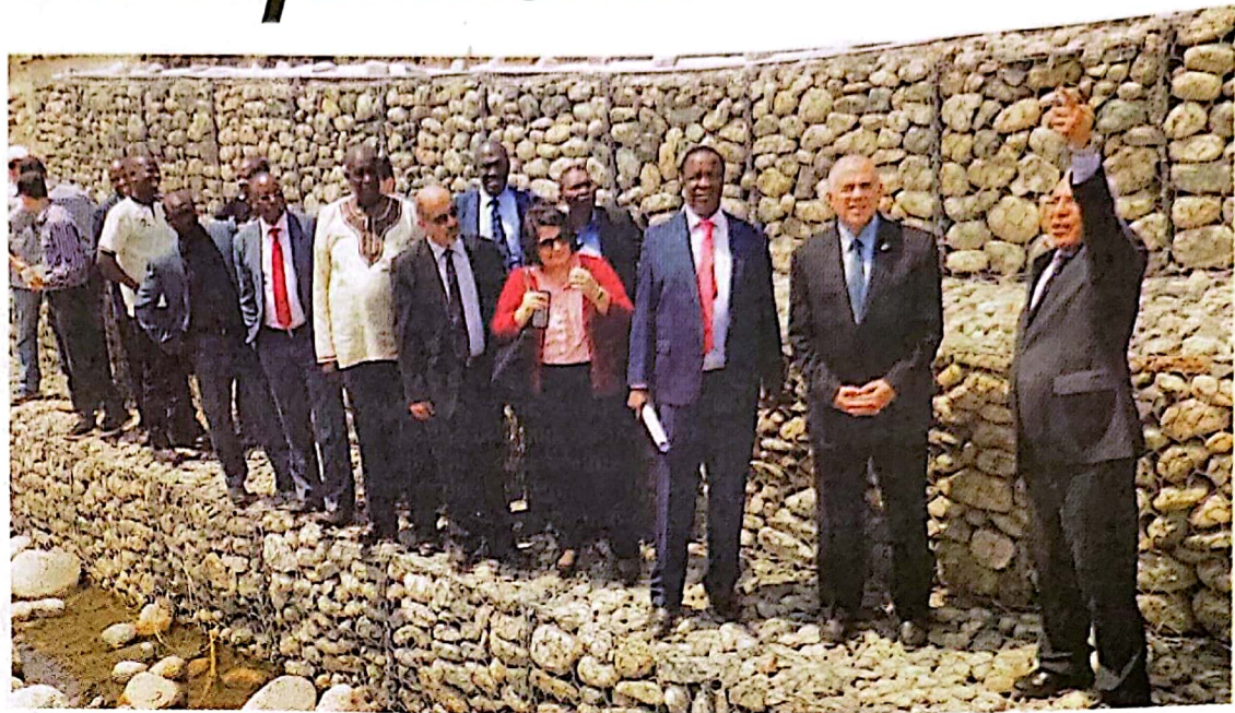
Officials of Arab Contractors taking quests on a tour of the gabions constructed near Road Barrier Primary School in Kasese district. Photo by John Thawite
