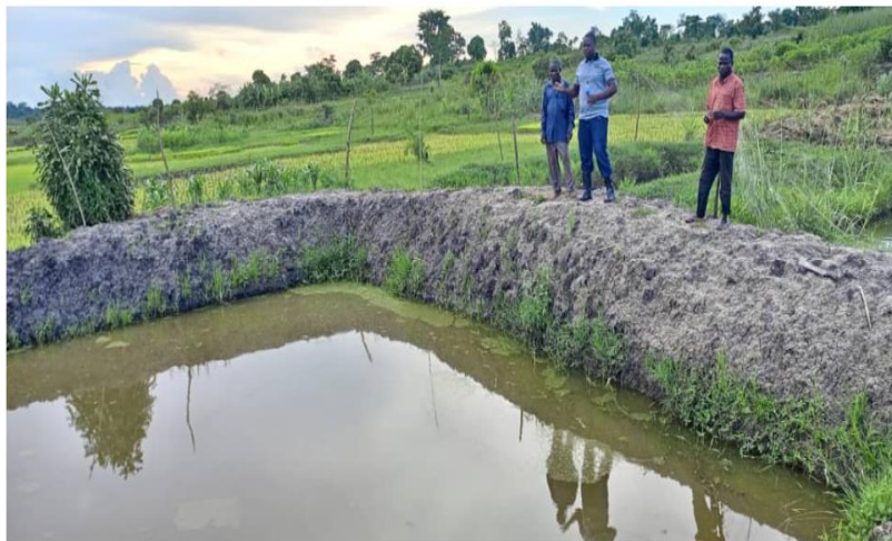
Plate 3. Minimising flooding by increasing banks on farmer's pond
