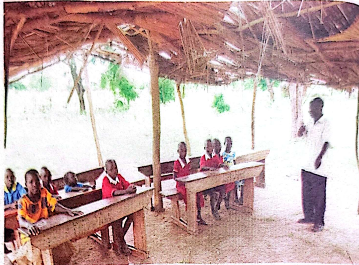
Structure. Pupils of Wairagala Primary School in Budaka District attend a lesson under a makeshift structure last week. PHOTO BY MUDANGHA KOLYANGHA
