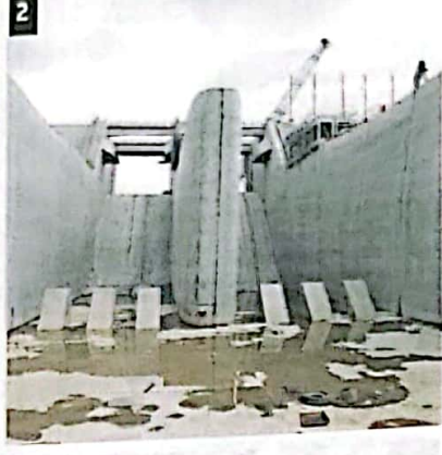
1. Concrete casting of the guide wall
