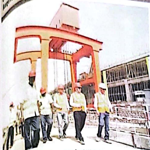
Tuning the upstream gantry crane installation
