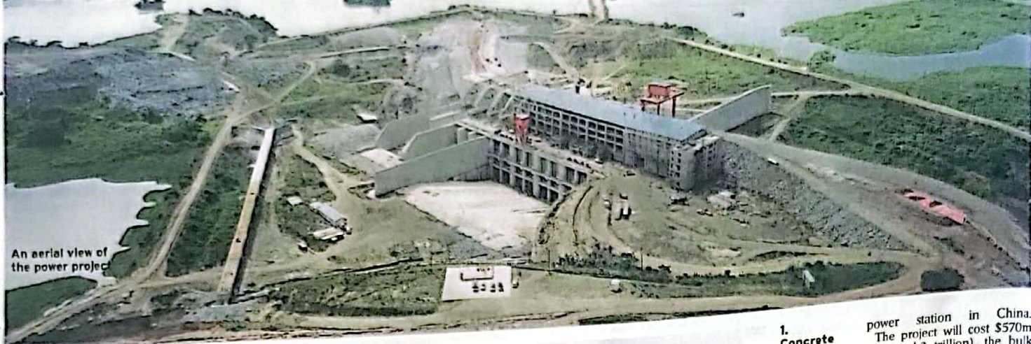
2. Concrete casting of the downstream apron Pictures by Richard Sanya
