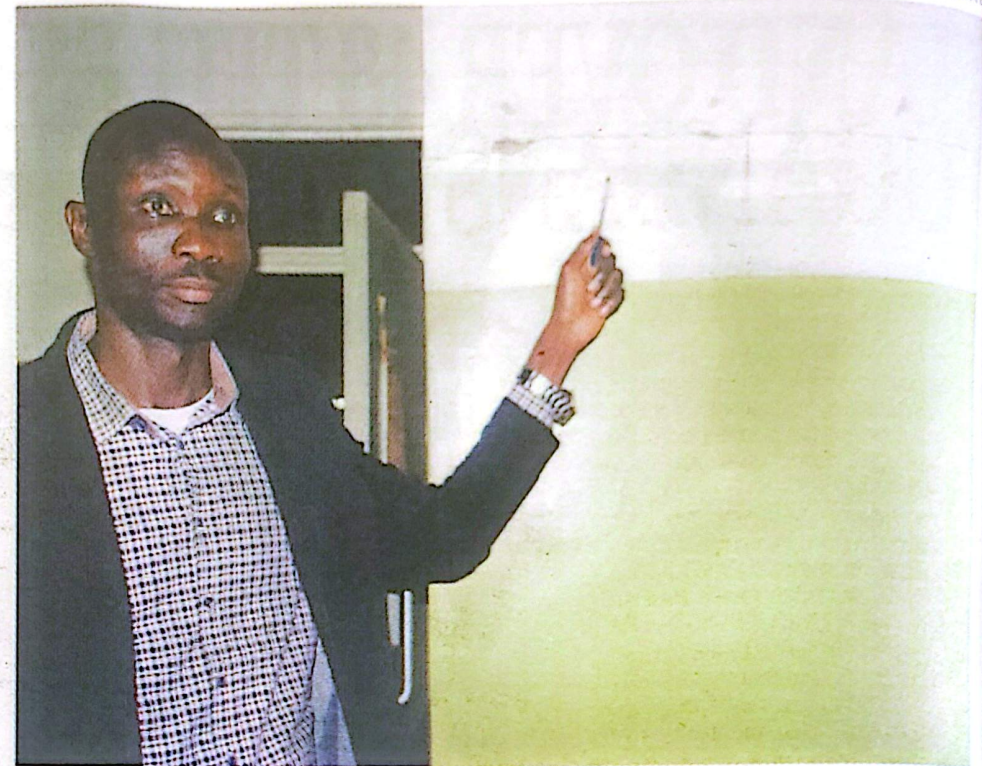
The administration block of Adjumani Hospital, which is cracking, requires renovation
