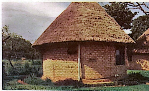
The exterior of the bandas which are used as accommodation units.
