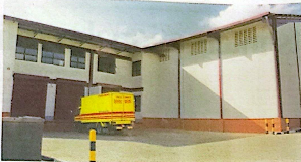
Prof. A.M Odonga warehouse in Kampala, Joint Medical Store's new facility in Kampala
