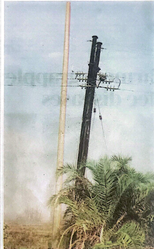
Some of the electricity poles that were recently erected after the previous ones were destroyed by bush fires in Awo Village, Bobi Sub-county, Omoro District in February 2021. PHOTO/TOBBIAS JOLLY OWINY
