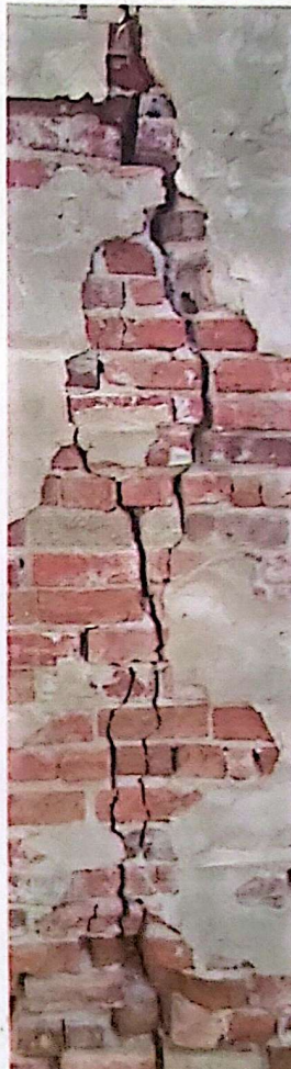
Using expansion joints in your brickwork will separate your bricks into small segments, in which, each segment will act individually, and will behave separately from other segments. FILE PHOTO
