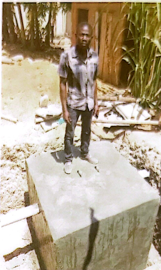
A man stands on top of a finished bio-digester. PHOTOS BY ROLAND D. NASASIRA
