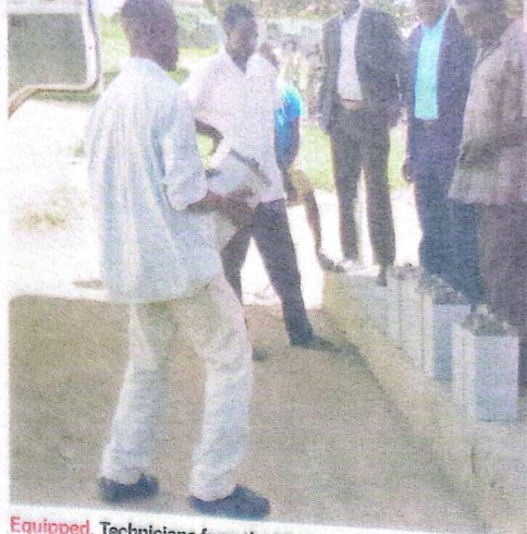
Equipped. Technicians from the Ministry of Health offload solar batteries and other equipment at Kamuda Health Centre III in Soroti District last week. PHOTO BY SIMON PETER EMWAMU
