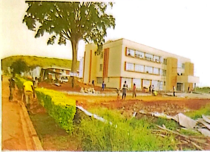
The University Lib. constructed under ADB project by PRISMA UG.Ltd
