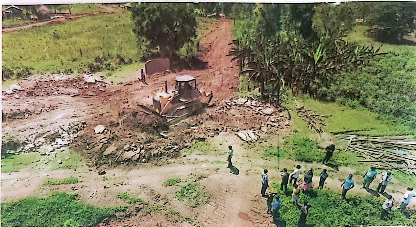
Preparation. A grader excavates land where the Standard Gauge Railway line is supposed to pass in Tororo District last month. PHOTO BY RACHEL MABALA
