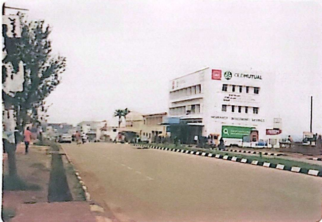
Mbale Republic Street under reconstruction
